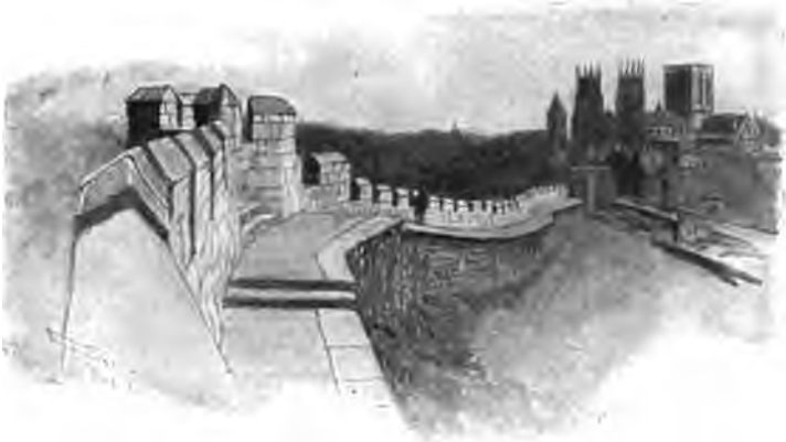
THE CITY WALLS OF YORK, ENGLAND
